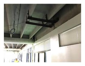
Structural Supports for Roof Openings
